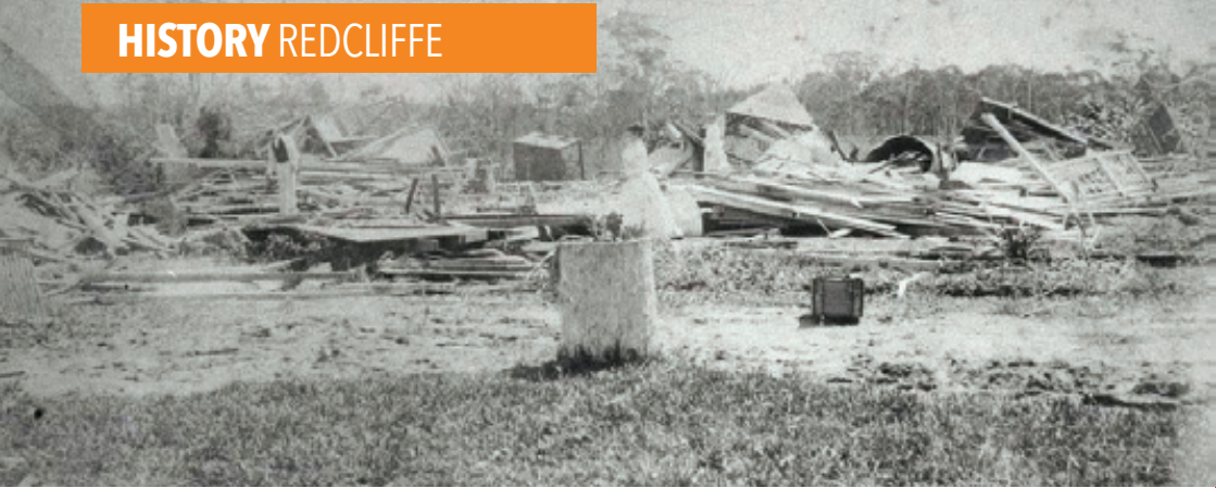
Mrs Bell's house, Klangur, destroyed by the 1893 cyclone
